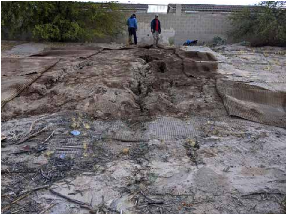
During an inspection of maintenance work in the Santa Rosa Wash, Maricopa Flood Control District director David Alley discovered a large-scale erosion problem created by a Senita homeowner backwashing a pool onto the upper bank of the wash. It cost more than $5,000 to repair and restore.
