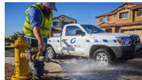
Global Water technician Scott Williams flushes a hydrant in Homestead.
